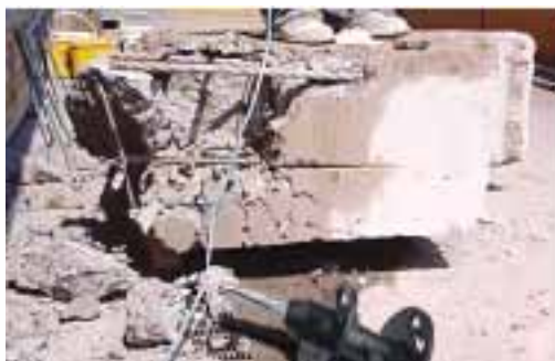
The Rock Cracker is also suitable for splitting reinforced concrete foundations, even inside buildings.
