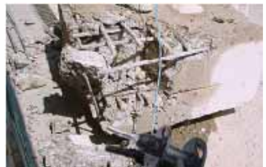
Heavily reinforced concrete can easily be split with the Rock Cracker.
