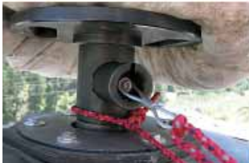
11 The pull rope is inserted onto the Rock Cracker.
